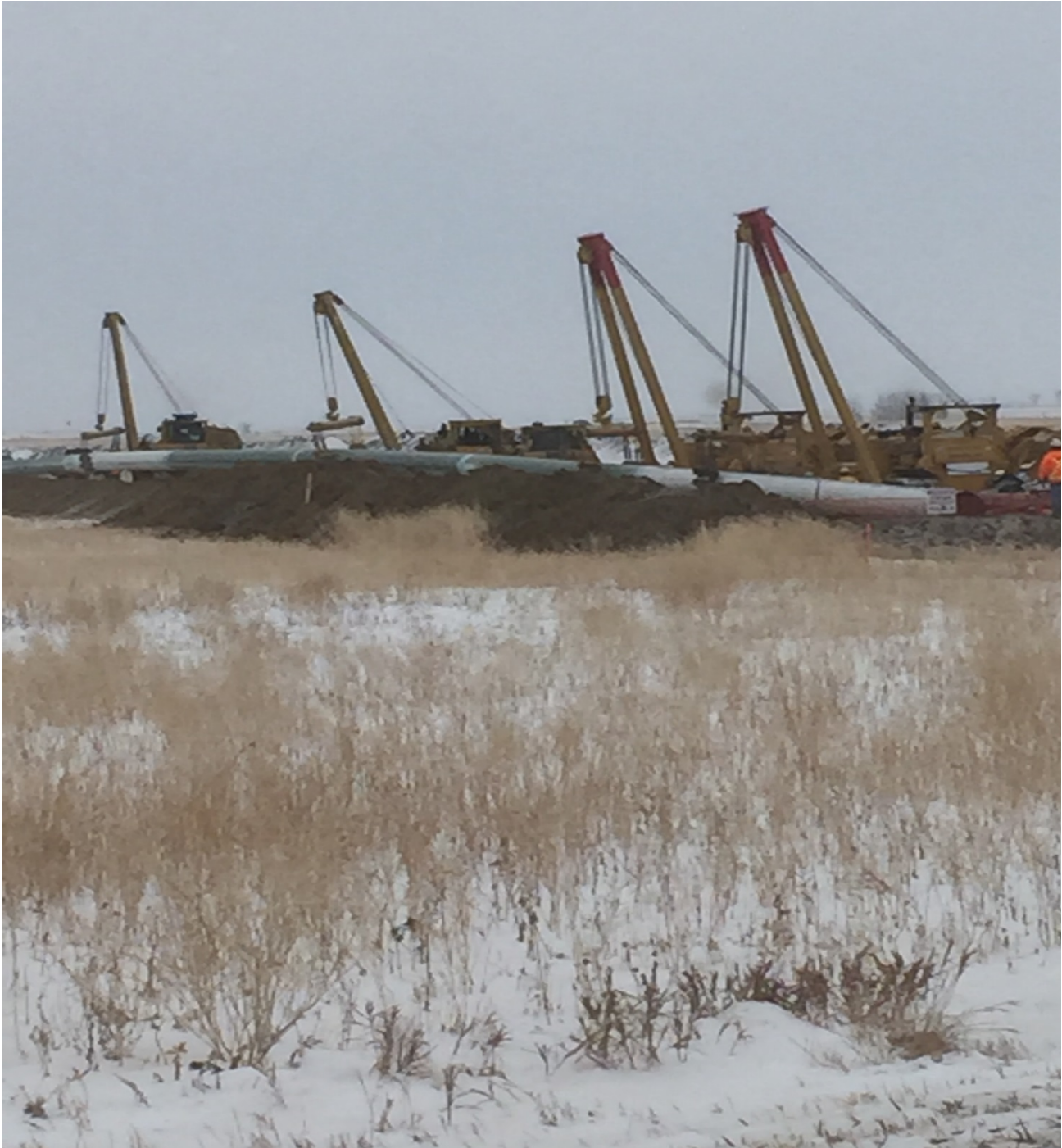
Laying the pipe into the trench
