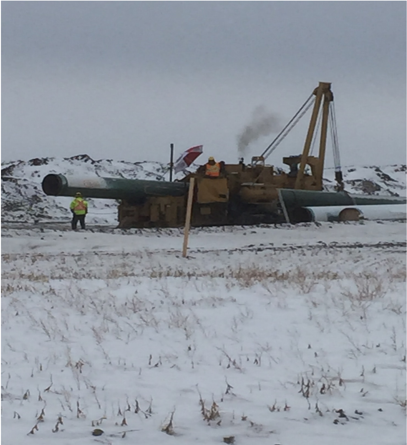
Pipe benders at work
