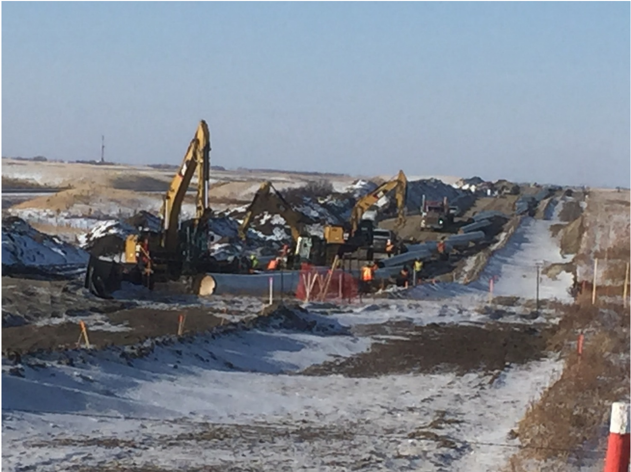
Pipe being strung on right of way
